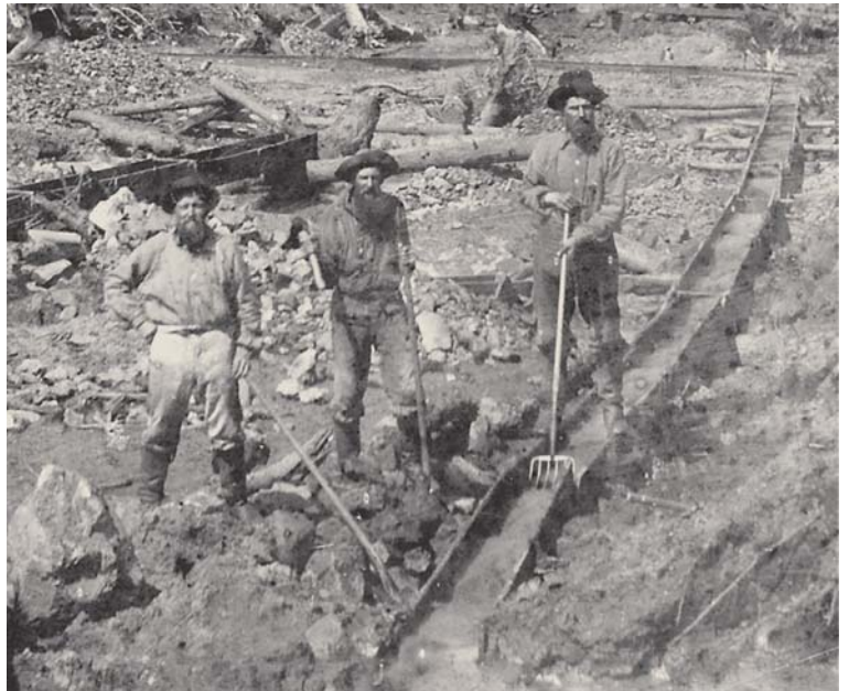
Placer Miners, circa 1865. The prospectors drawn to the Gregory Diggings in search of riches first worked the surface. They panned for gold in streams, then they built sluice boxes and flumes.
