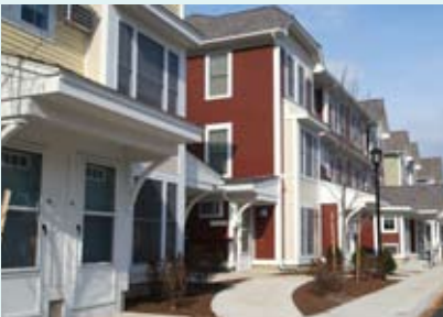
Olmsted Green A bank-supported affordable housing project
